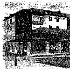
LSU - New Residence Hall - Phase 2 Estimated Completion: Owner: State of Louisiana Cost: $25.2 Million - 115,000 SF Location: Baton Rouge, LA
